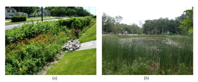
**Figure 5:** Infiltration trench (a) and Phyto-purification basin (b). *Source: Aaron Volkening, [CC BY 2.0]. Retrieved from Flickr.com.*
