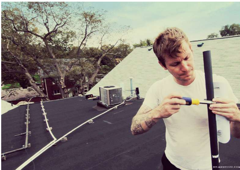
Fig. 2 - Andrew Reynolds, from the development team that landed a software to operate Detroit MESH network, installing a relay mast. Screenshot taken from “48217 Mesh” by Nora Mandray and H el ene Bienvenu –   Nora Mandray (2013) – www.diy-manifesto.com.
