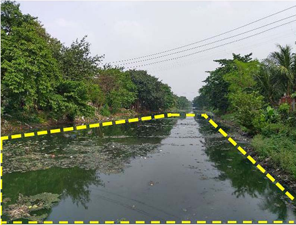
Fig. 7: The contaminated condition of the canal. (Source: Taken by author)
