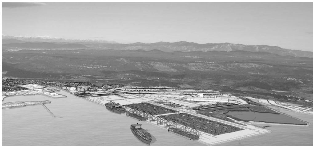
fig.6 - View of the Monfalcone Port Project
