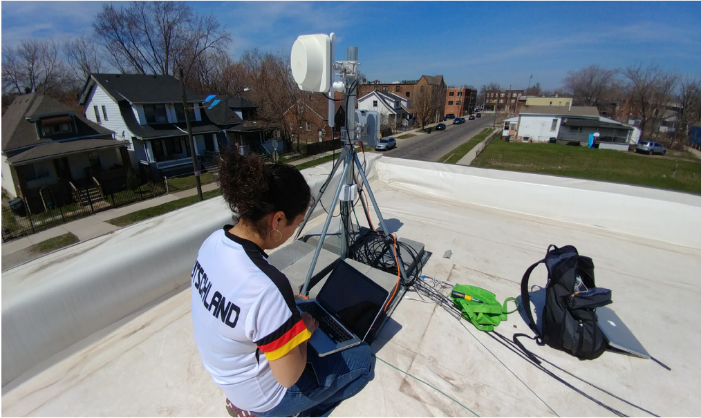
Fig. 3 - Digital Steward assembling and checking a MESH antenna – © Detroit Community Technology Project – Allied Media Project – https://detroitcommunitytech.org/
