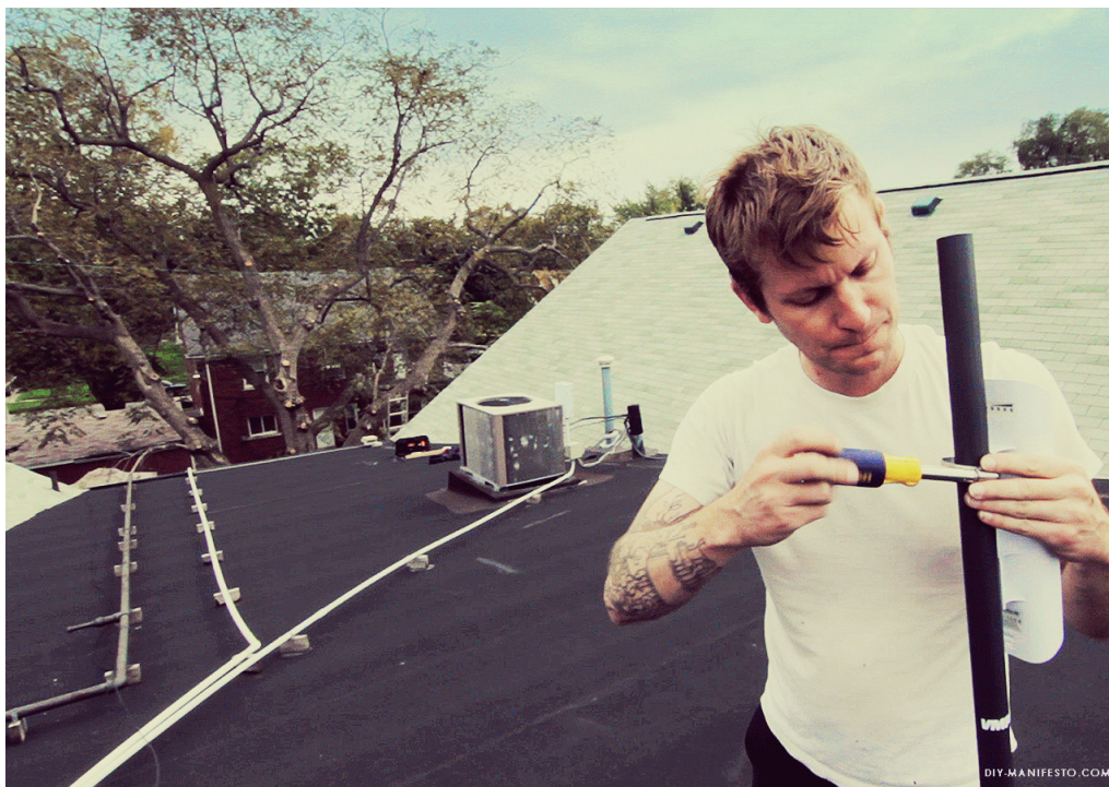
Fig. 2 - Andrew Reynolds, from the development team that landed a software to operate Detroit MESH network, installing a relay mast. Screenshot taken from “48217 Mesh” by Nora Mandray and H el ene Bienvenu –   Nora Mandray (2013) – www.diy-manifesto.com.
