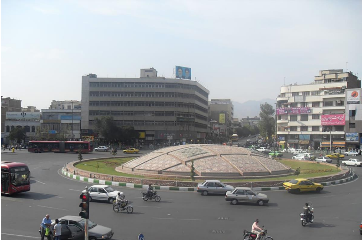
Fig. 7 Enghelab Square is one of the main nodes of Tehran, under which a metro station was established in 2009
