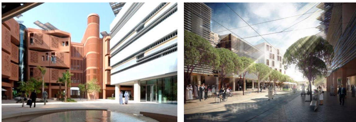
Fig. 5 - 6 Central Courtyard of the Masdar Institute Campus (left) and Central Spine Showing Light Rail Transit and Retails -artist impression (right)
