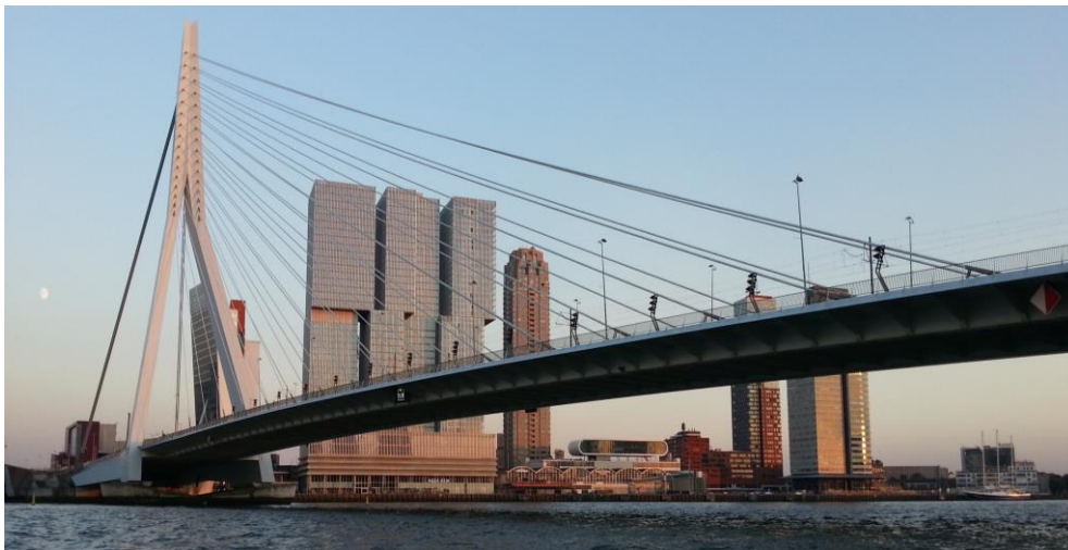
Fig. 10 – Kop van Zuid today. View from the river, Rotterdam 2018
