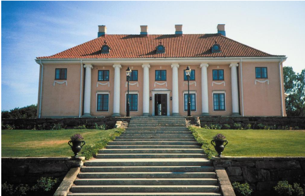
Fig. 1 – The Rossared Manor
